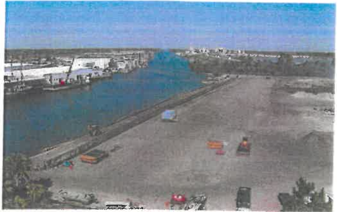
Photo 1. Bulkhead Improvements on the Gulf County Canal, Port St. Joe
